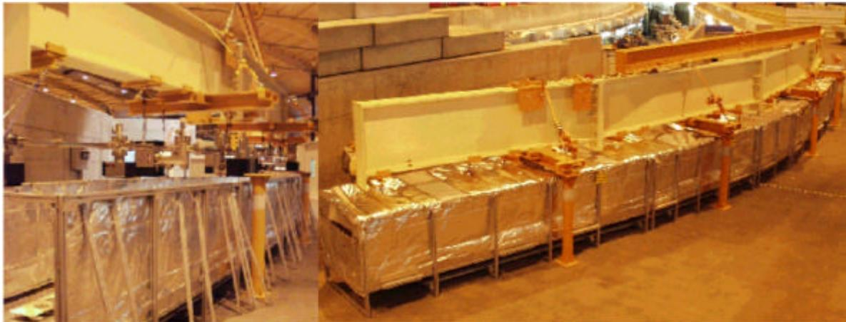
Fig. 5a SLS vacuum section on the way into the bake-out tent
